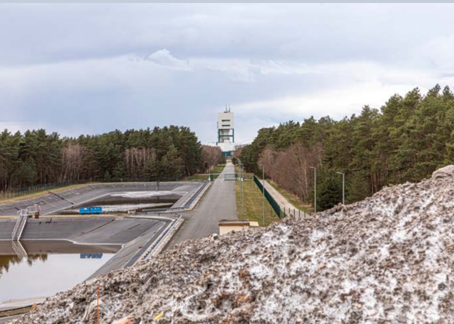
Gorleben mine: Dismantling has begun
