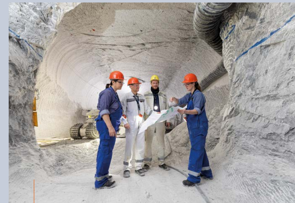
Morsleben repository: Demonstration structure in the main anhydrite
